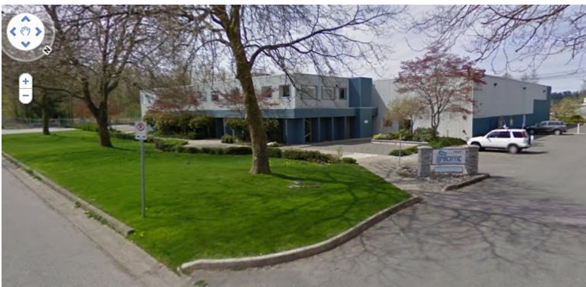
Figure 9: PCC Front Entrance
